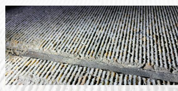
concrete as traffic driving over a textured surface emits less noise than when driving over a smooth surface.
