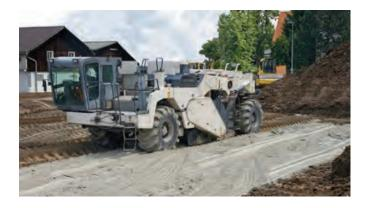
CalBlend immediately dries up fine clay containing soils. It also improves the working conditions during construction, thanks to the flocculation effect of lime and clay. Cemblend can also provide Geotechnical pre-studies that can optimise the reuse of soil, resulting in long-term improvements.
